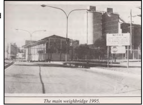
The main weighbridge 1995.
