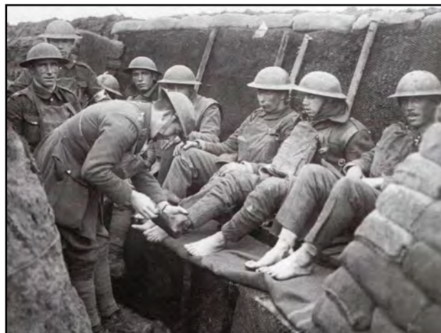
Soldiers in a trench having their feet inspected for Trench Feet
