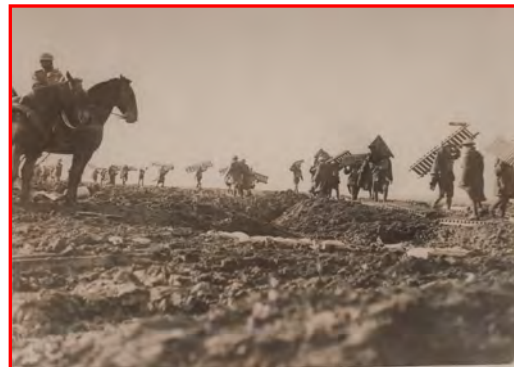
Pioneers laying a duck board track through craterfield 5/10/1917.
